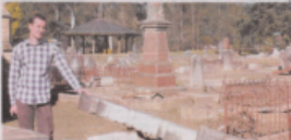
While St Mark's church is open for services, the cemetery is the next fix-it project after the Pickett storm event in June 2016 damaged the church building and historic graveyard.
